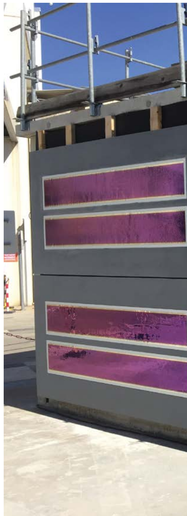
By combining a PV facade system and precast concrete panels, a building will be able to generate much more solar energy.
